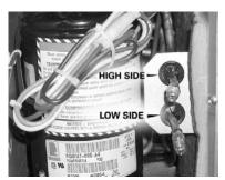
Figure 11: Schrader connections
